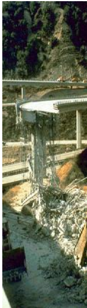
LA freeway after 1994 Northridge earthquake
