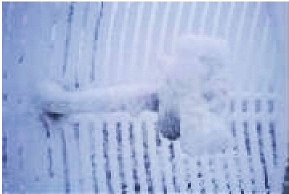
Fig. 8. Snow and ice on a grid antenna at the La Jolla relay
