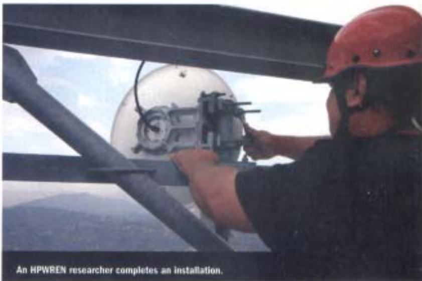
Earth scientists set up a communications node to transmit data from sensors that measure the strength of earthquakes in Anza Borrego Desert near Borrego Springs, Calif.
