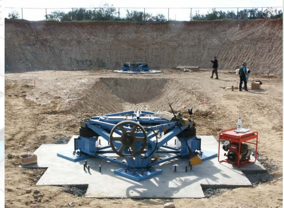
Shakers in LHPOST Reaction Mass Pit
